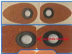
INCORRECT OVERLAP - TAPE CANNOT OVERLAP THE METAL RINGS THIS WILL CAUSE LEAKS.
